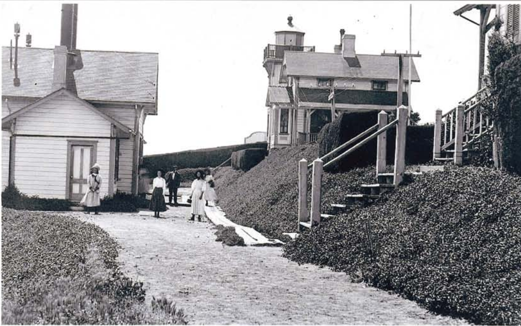
247 C. Conant 210 Beach Avila Beach, Calif. 1910 Old light house, buildings
