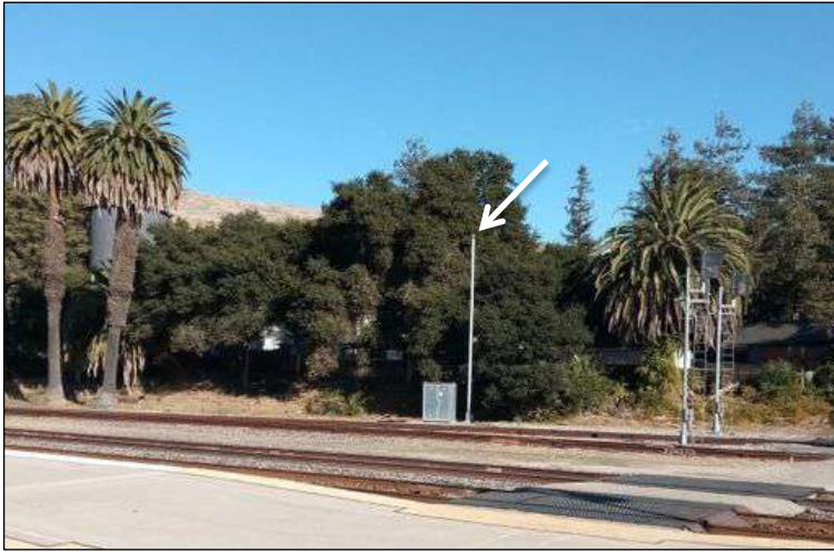
San Luis Obispo's special blue light (white arrow) stands tall, with signals controlling exit from the Amtrak layover track and the pocket track for helper locomotives to the right, and the historic water tank and palm trees to the left.
